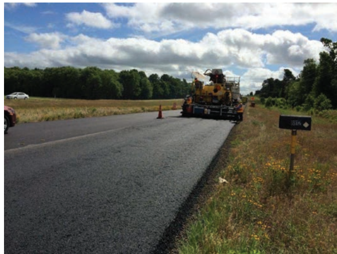
Figure A.12: Observed Segregation Even after Increasing the Production Temperature.
