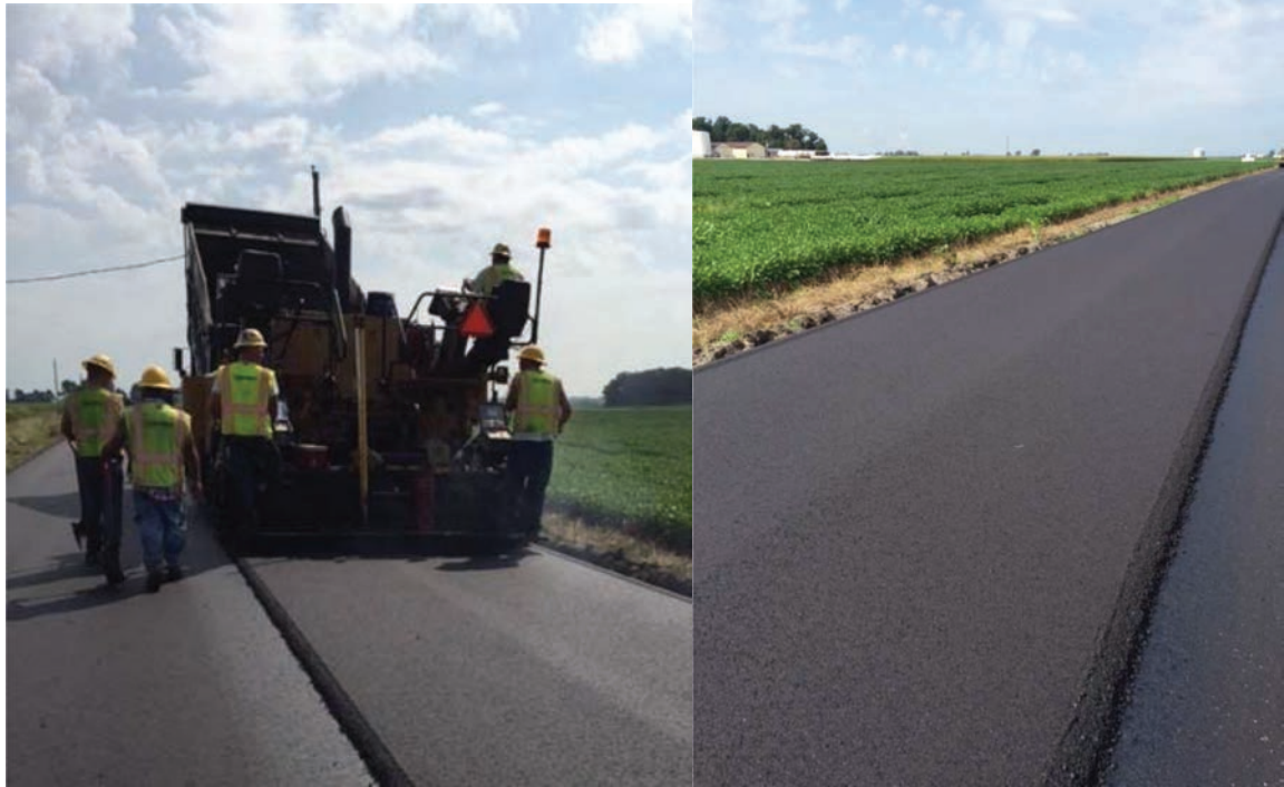
Figure C.11: Paving of the surface layer at the Indiana field project.
