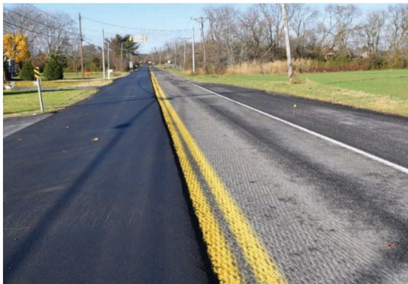
Figure E.1: Project Site showing Surface Course and Milled Surface.
