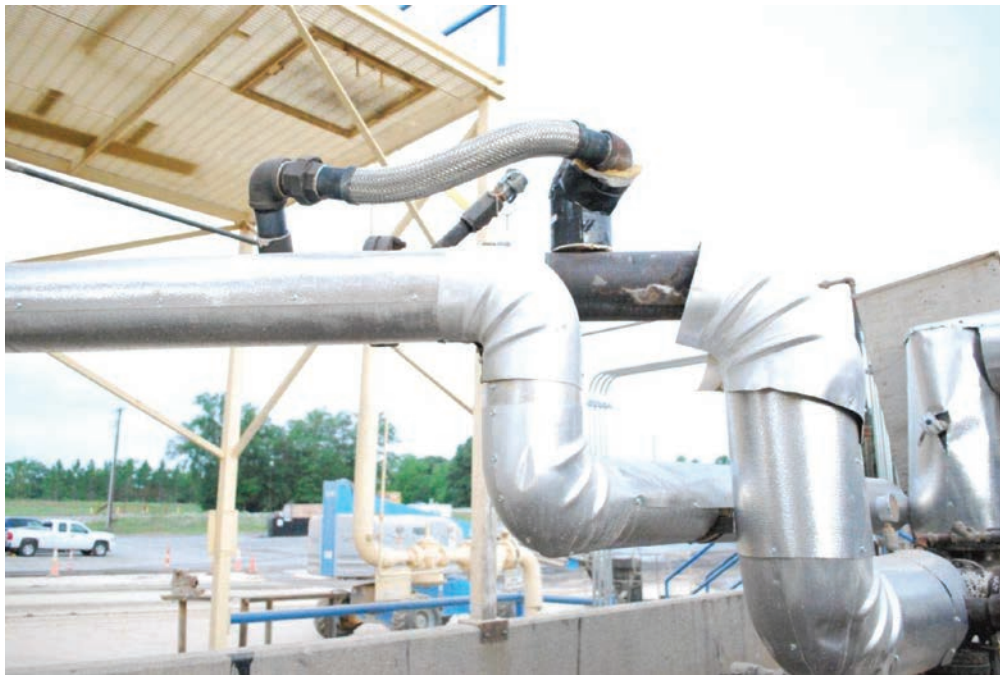
Figure A.17: Admixture/Rejuvenator Injected Directly into the AC Line.
