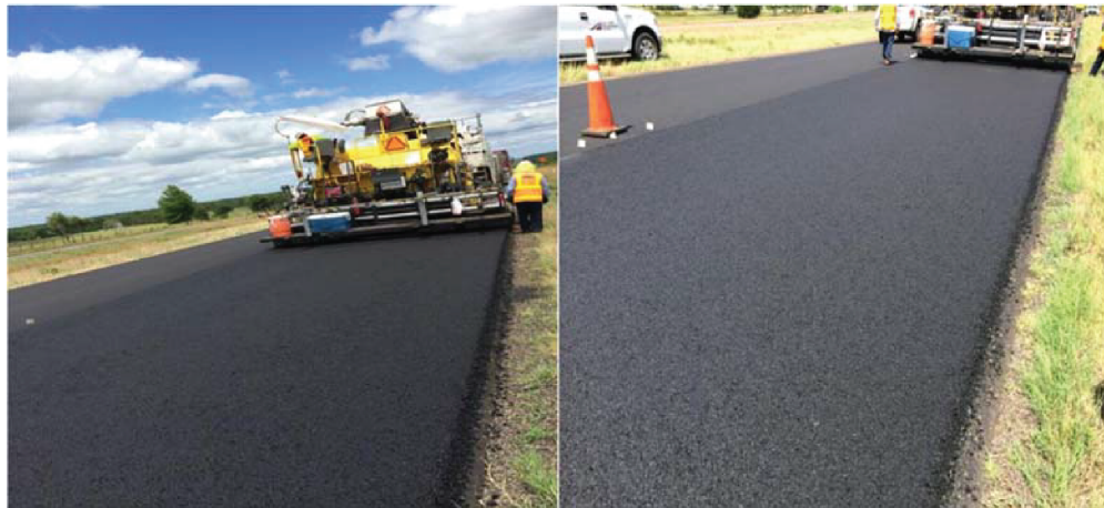
Figure A.13: No Obvious Segregation in Section 5.
