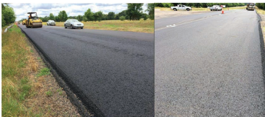
Figure A.8: Section 2; (a) Observed Segregation on Loose Mat, and (b) Finished Surface.
