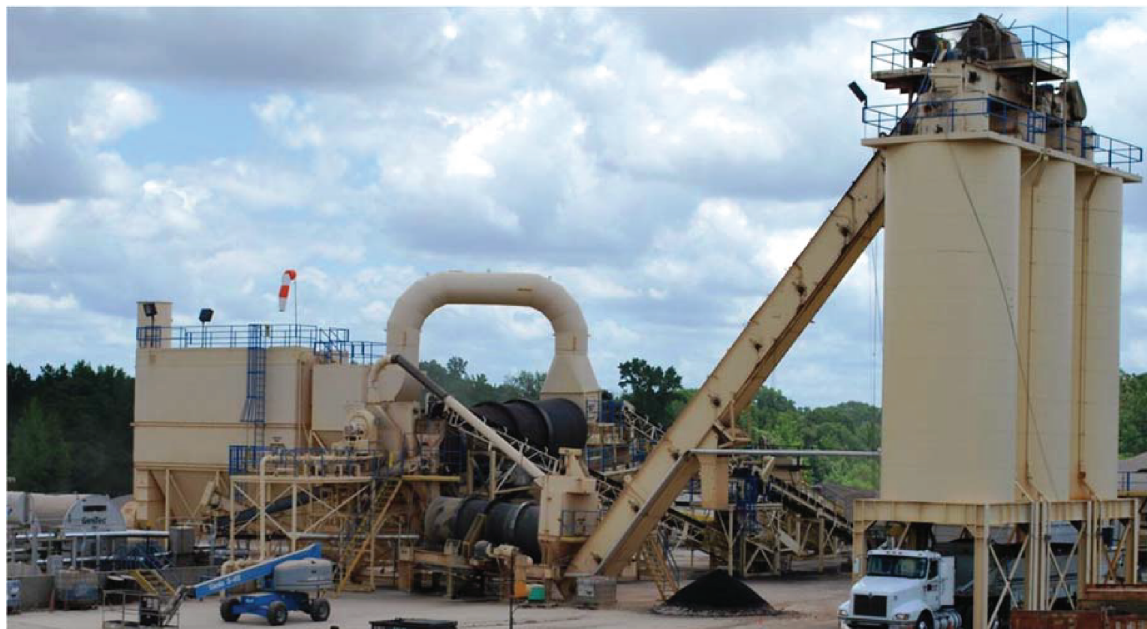
Figure A.14: Overview of the Asphalt Mix Plant.
