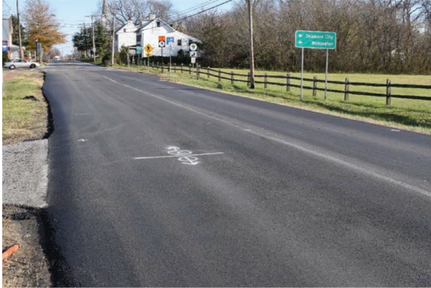
Figure E.12: Finished Pavement Surface.
