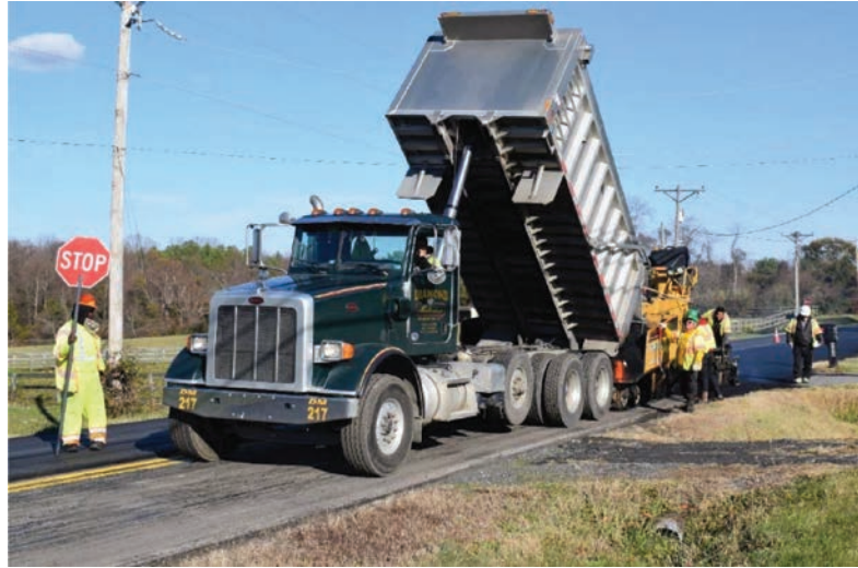
Figure E.10: Paving of the Surface Layer.
