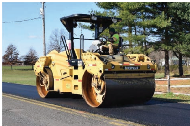
(a) Vibratory Roller
