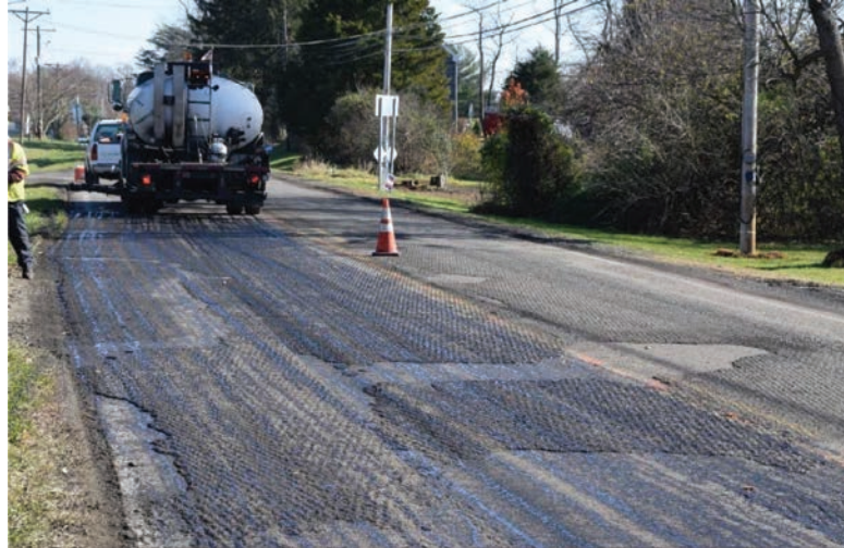
Figure E.9: Application of Tack Coat on Milled Surface.
