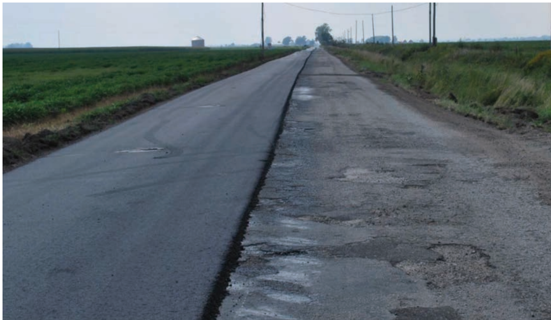
Figure C.2: Binder course and existing pavement surface at the Indiana field project.
