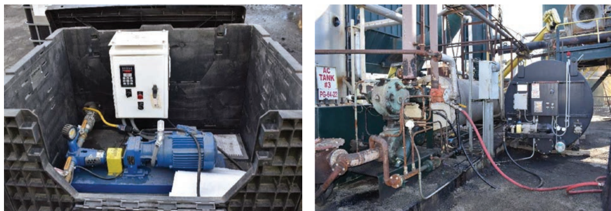
Figure E.8: Injection System of the Warm Mix Additive and Recycling Agent to the Binder Line and Pump to Regulate Rate.
