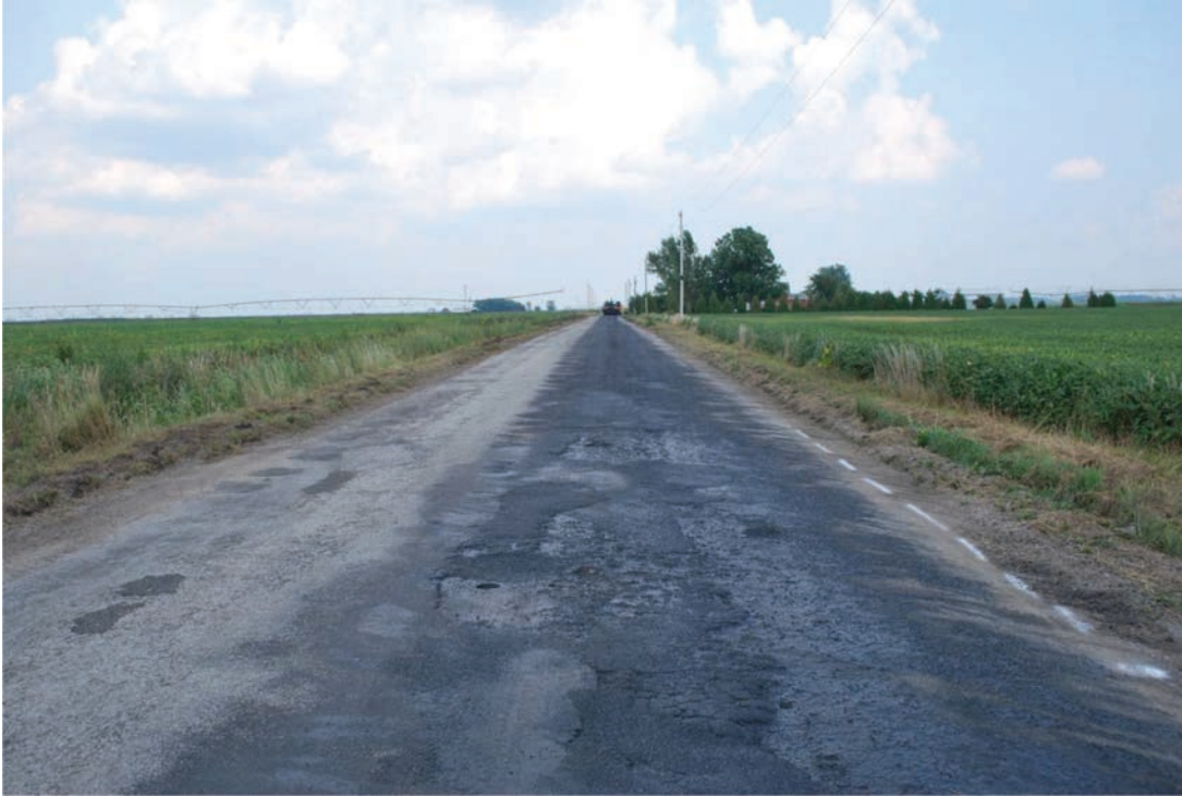
Figure C.3: Existing pavement surface at the Indiana field project.
