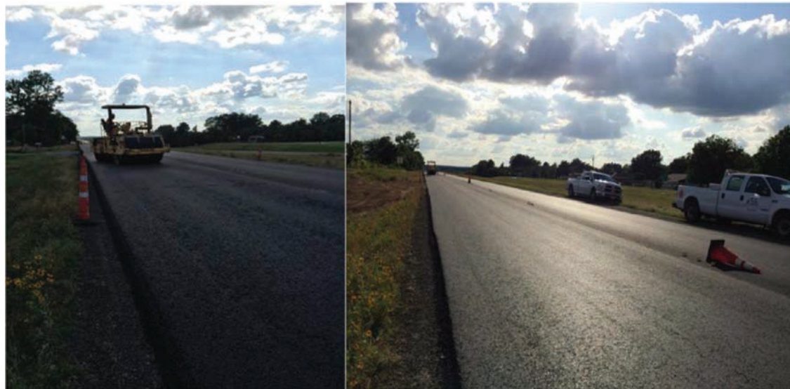
Figure A.9: Section 3; (a) Observed Segregation on Loose Mat of Section 3, and (b) Finished Surface.
