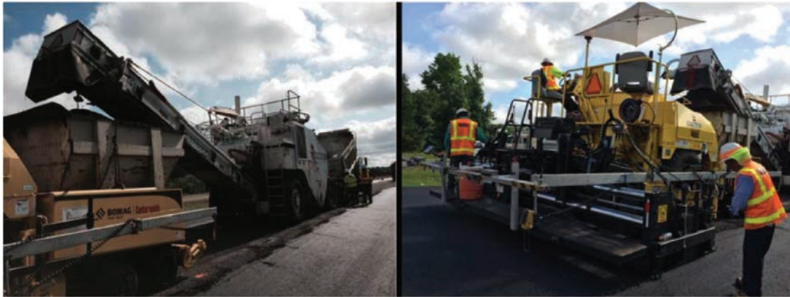
Figure A.5: Shuttle Buggy and Paver.
