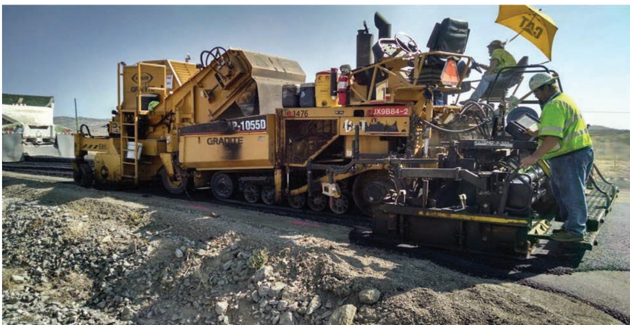
Figure B.5: Picture of the windrow lifter and paver.
