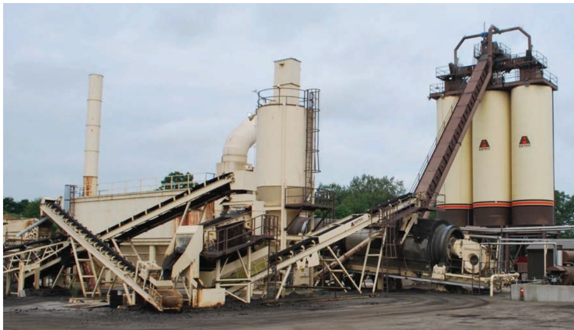
Figure C.9: Overview of asphalt mix plant at La Porte, Indiana.
