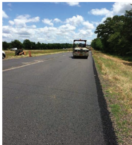
Figure A.7: Finished Test Section 1: Virgin Mix.
