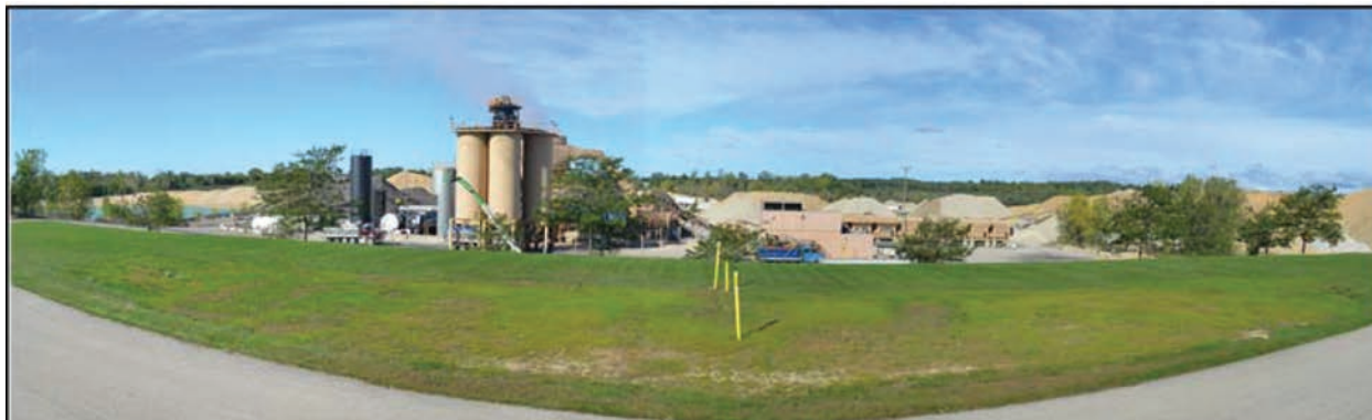
Figure D.3: Asphalt Plant Overview.
